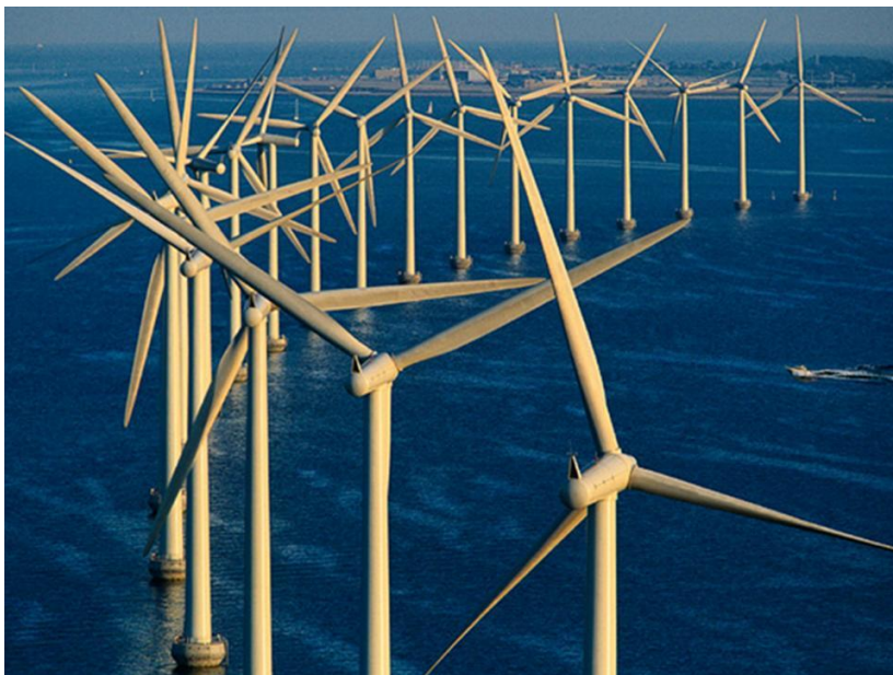
Fig.1 – Example of installations.
